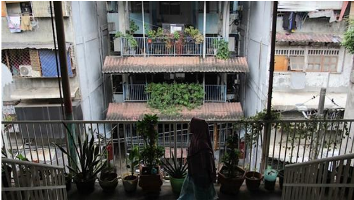
Figure 2. Existing Conditions of Kebon Kacang Flats, Central Jakarta
