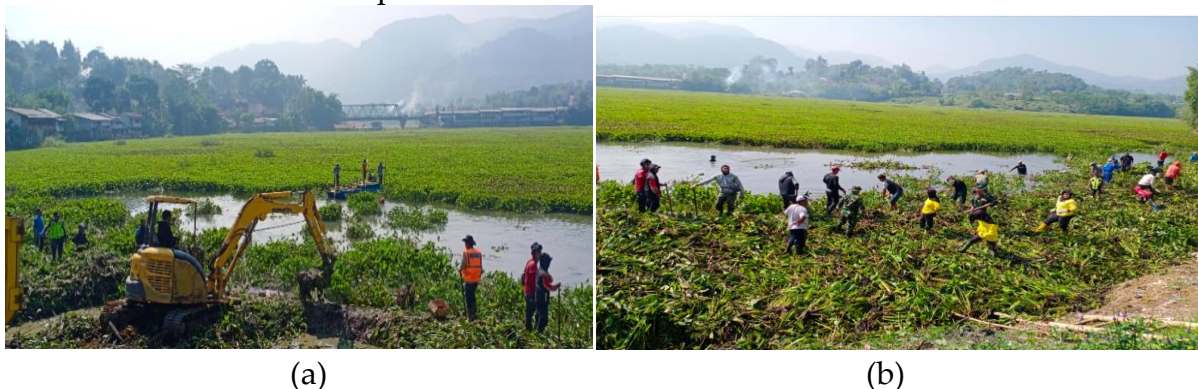
Figure 4. Removal of Water Hyacinth At Saguling Reservoir Using an Excavator (a) and Manually (b)
