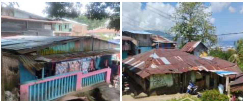
Figure 1. Condition of residential buildings
